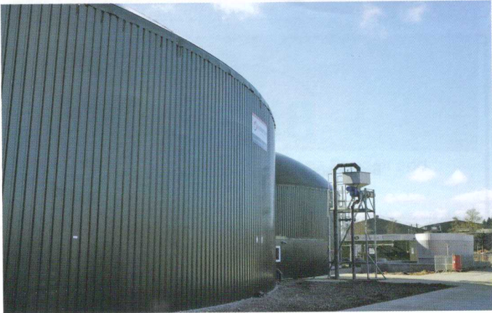
The recently completed anaerobic digester.
